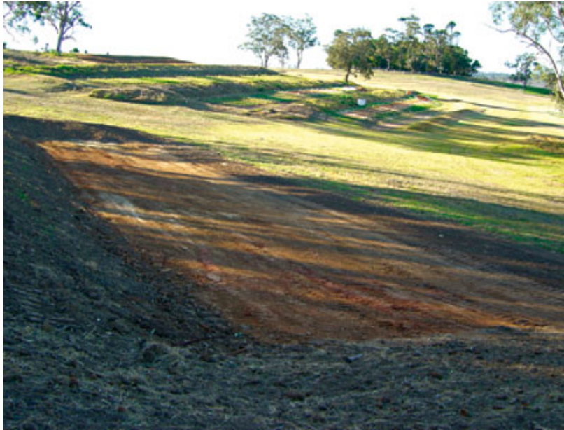
Figure 23. Area of CROA where vegetation and topsoil has been removed in preparation for the establishment of runoff plots (Block 1). Note the proximity to Blocks 2-4 and previous runoff plots established at the site.
